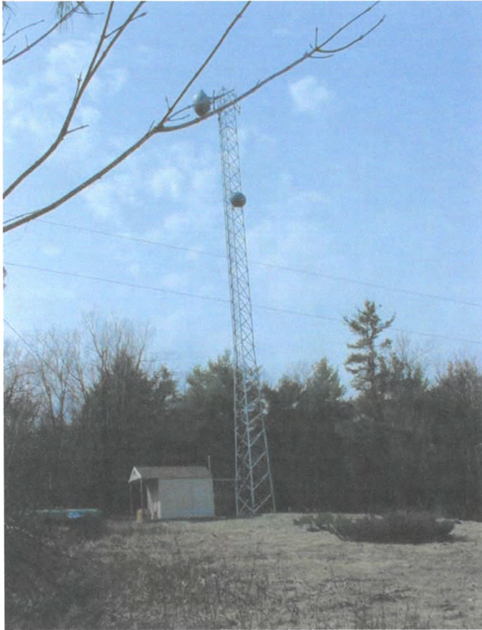
Cell tower located at the north end of Field # 3 Compartment III photo taken Spring 2006
