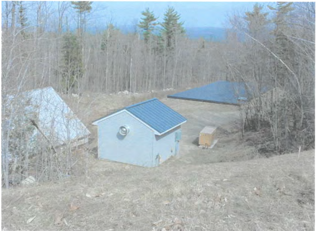
Well house complex that supplies water to the County Farm and Ossipee Village photo taken Spring 2006
