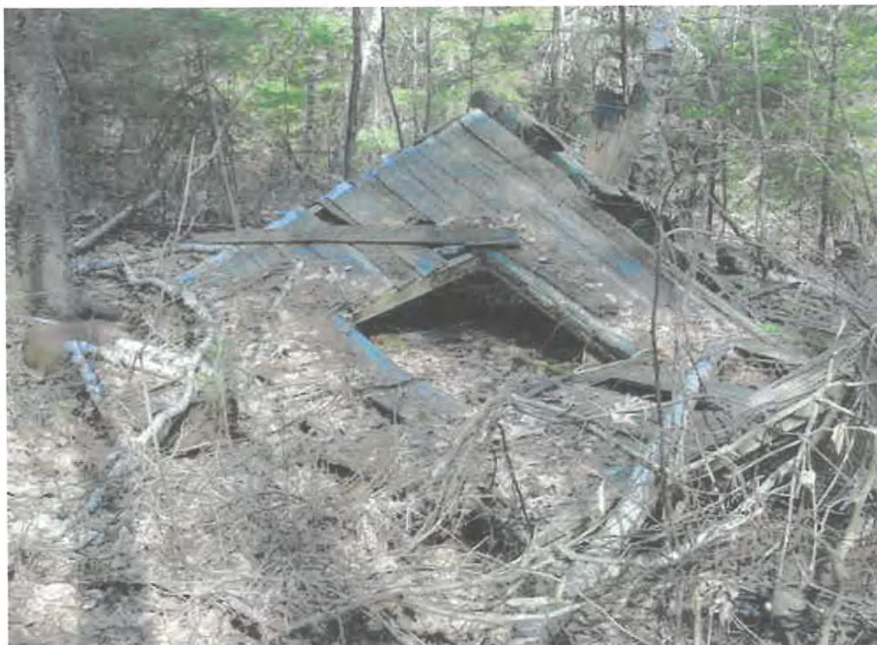
Remains of building at top of the ski slope photo taken Spring 2006
