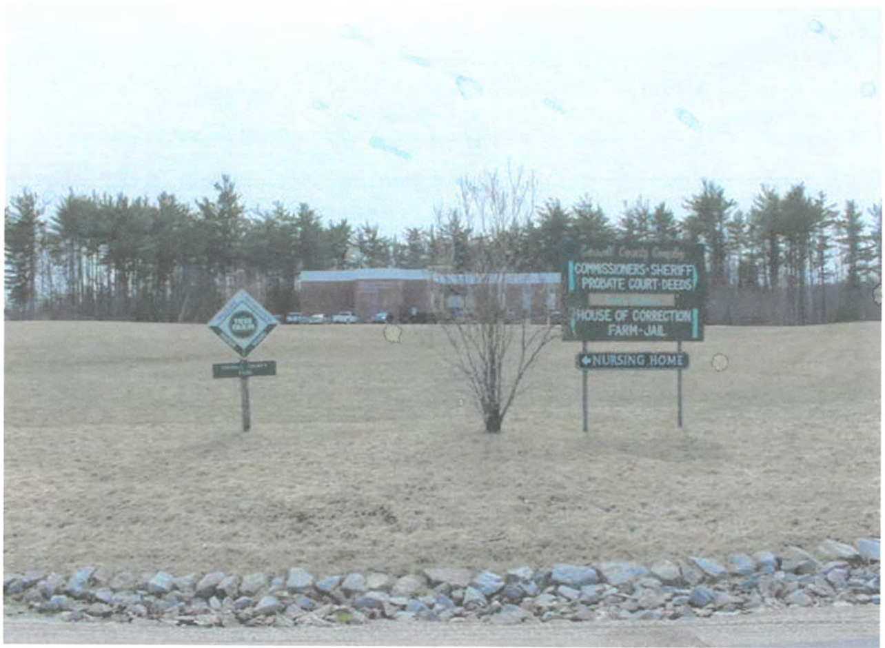
County Administration Building photo taken Spring 2006
