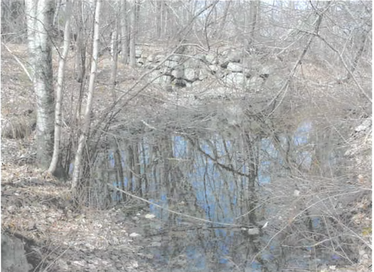
Barn Foundation adjacent to cellar hole photo taken Spring 2006
