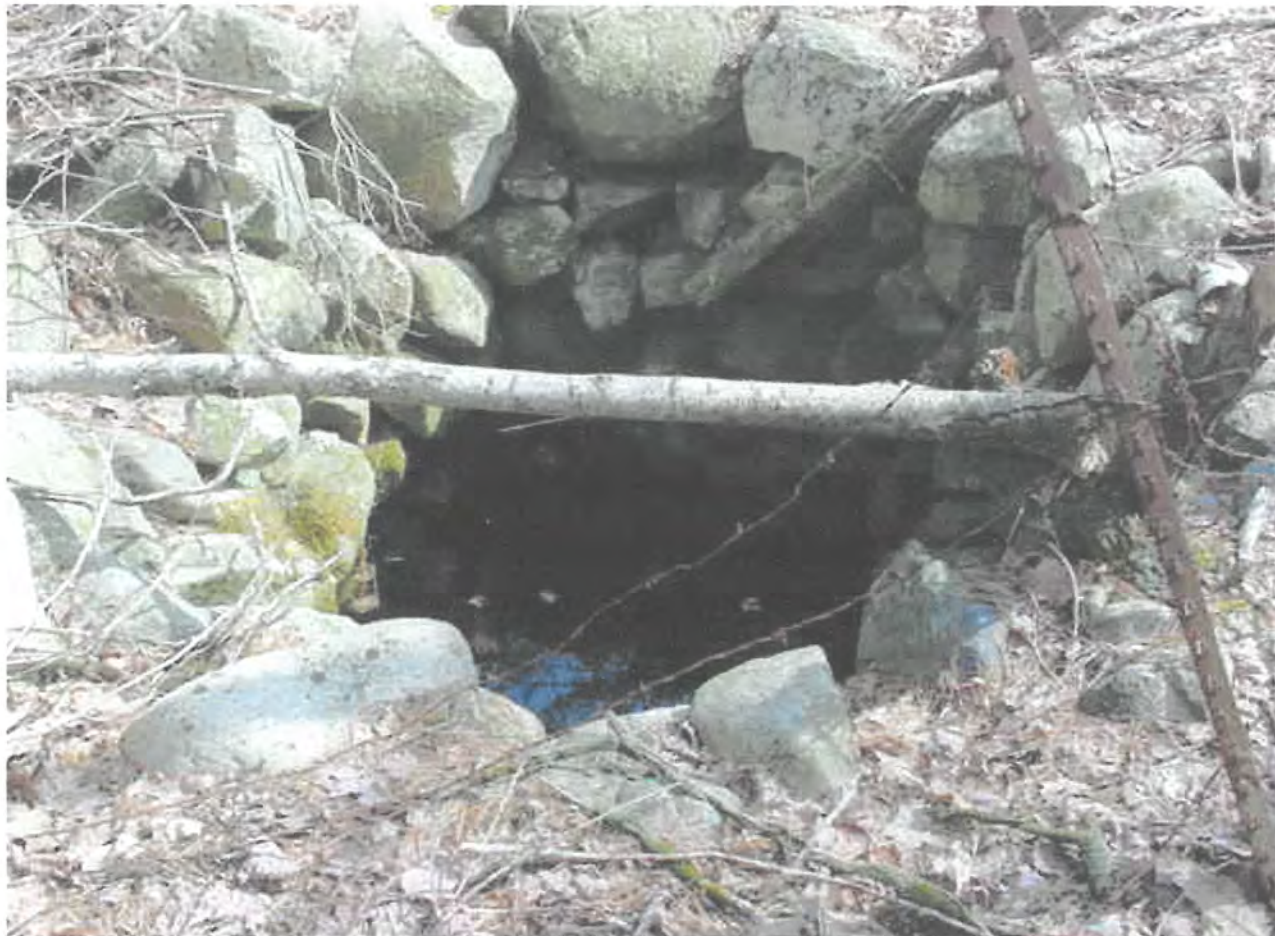
Open stoned well poses safety hazard photo taken Spring 2006
